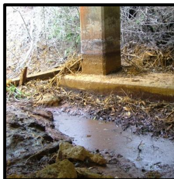
Concrete cancer from acid waters.
