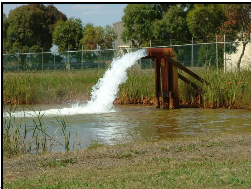
Extracted groundwater being delivered to the holding ponds at the Barwon Downs Borefield.
