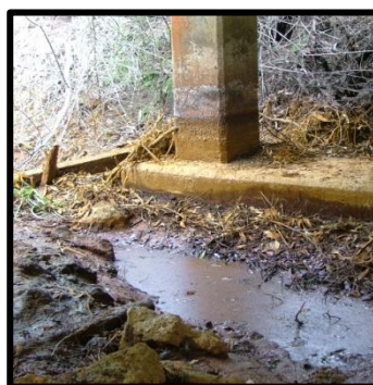
Concrete cancer from acid waters.
