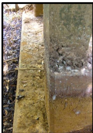
Concrete cancer from acid waters.
